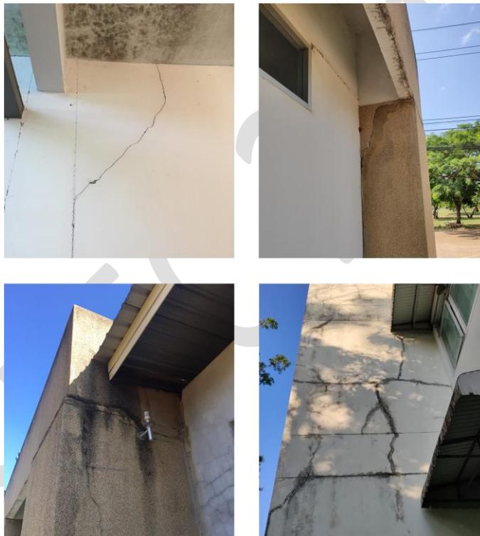
**Figure 12 Structures cracks on the building inside KU CSC due to the settlement.**
